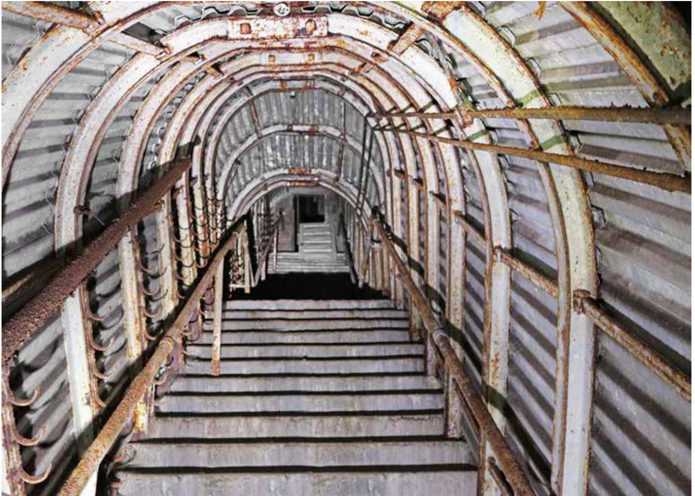
Looking up the steep eastern steps (179 steps) down into the WWII underground combined headquarters at Fort Southwick. The depth of the underground HQ varied according to the slope of the hill, but was in the region of 80-100 feet. Photo Clive Holden
